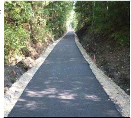
Constructed Section in Derry
